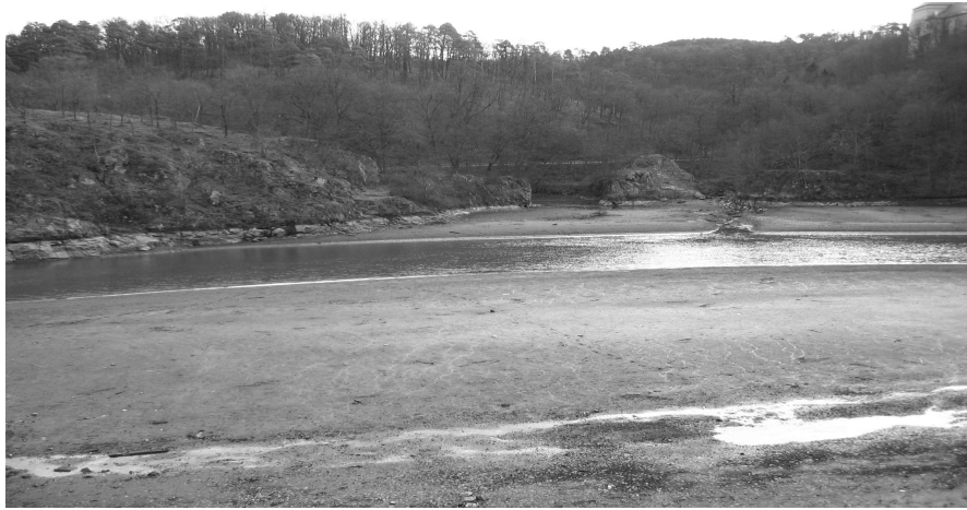
Fig. 4) The sediment on the reservoir bottom appears when the level of water is reduced
