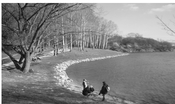
Fig. 1) Bank stabilization – Brno damm (foto M.Šlezinger, 2008)
