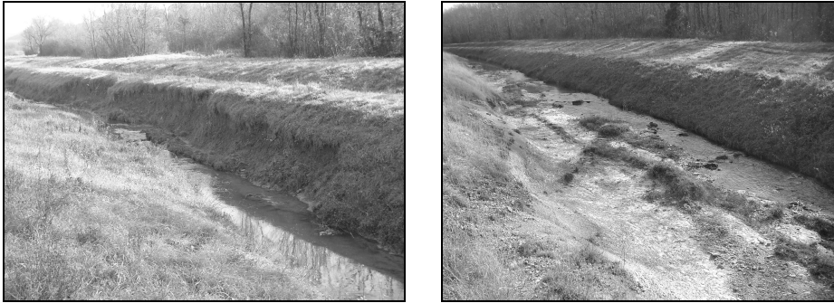
Fig. 3) Water erosion influence on mild curves of the Botonega Channel
