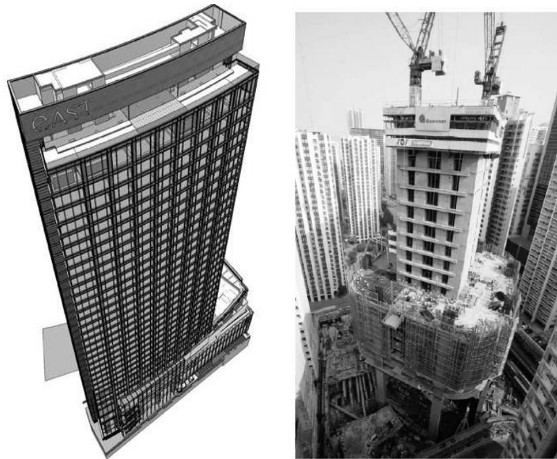
Fig. 1) The OIE project – BIM model output ( left ) and actual construction ( right ).
