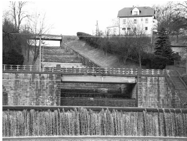
Fig. 1) Upstream view on stepped spillway of the Bystřička dam (taken by Povodí Moravy, s.p.).
