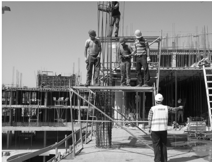
Fig. 2) Improperly made scaffoldings
