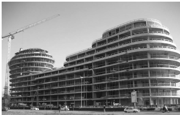
Fig. 1) Construction of residential – office building ACC
