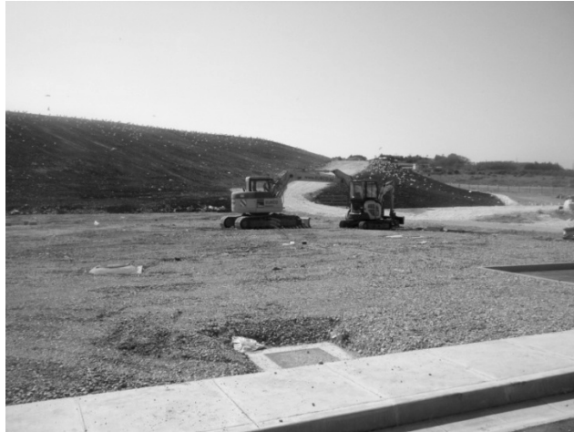
Fig. 5) Kaštijun landfill during remediation
