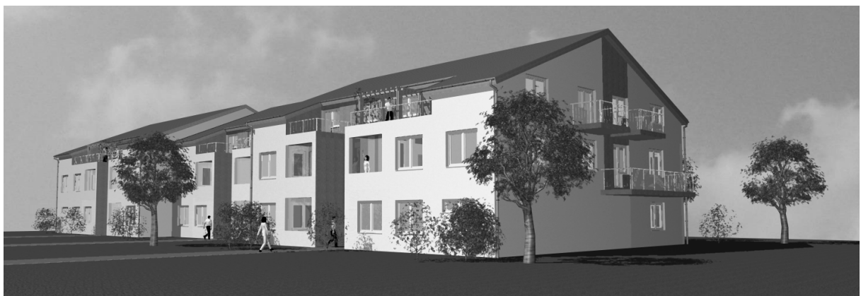
Fig. 2) View of apartment house consisting of three sections.
